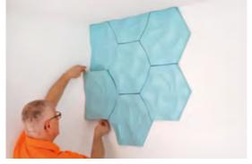
Professionally grout the ceiling and wall connection area with ADEFIX <sup>®</sup> adhesive filler if necessary.
