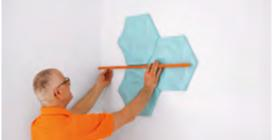
Measure the wall and establish the position of the ARSTYL® WALL TILES. Set out the lower laying line using a spirit level.
