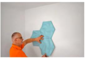
NOTE: Butt joint areas must not be glued or grouted.
