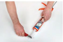
Clamp the adhesive cartridge, cut cartridge nozzle (diameter 5-8 mm).
