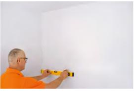
Set out the lower laying line using a spirit level.
